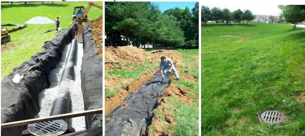
Figure 4: Example of Infiltration Trench Installation
